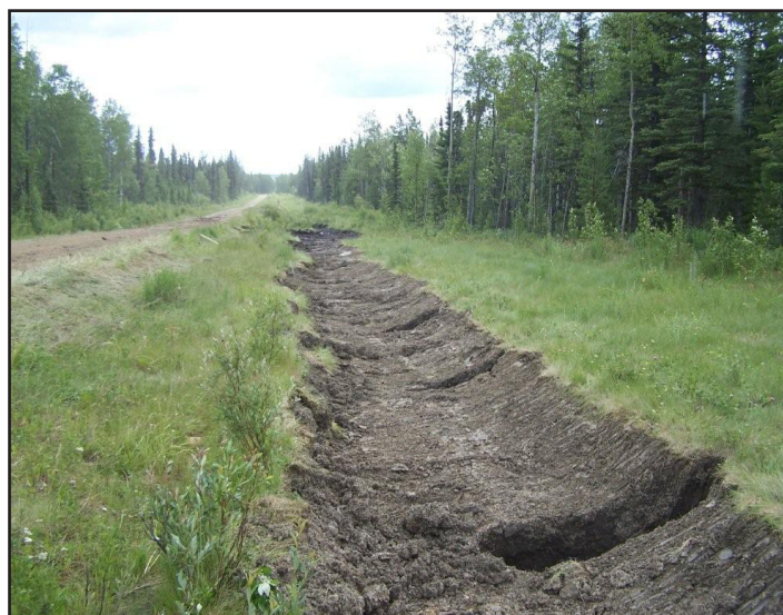
Hydrovac line exposure and excavation of contaminated material near Blackhawk Lake (2008).
