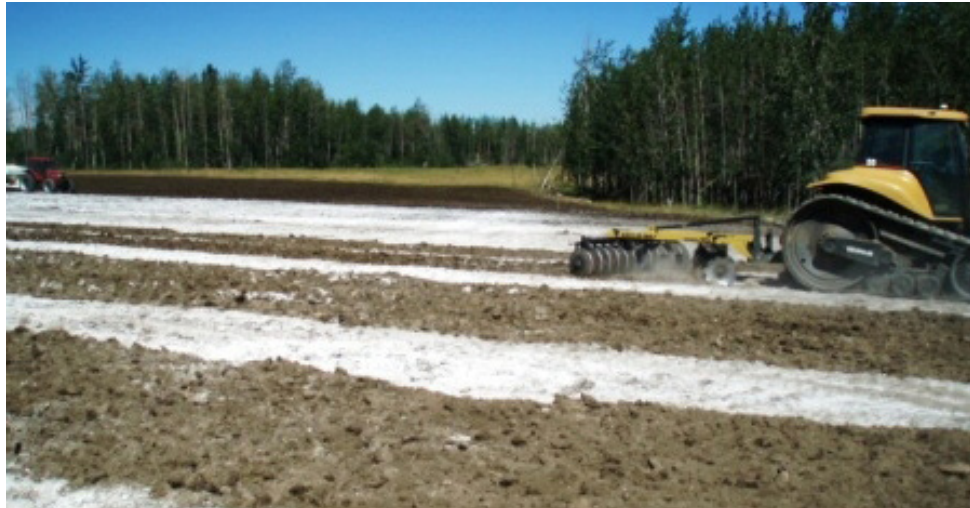
Using lime in the reclamation process
