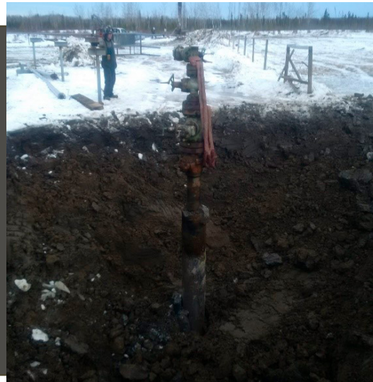
d-027-J/094-A-10 Well was plugged, cut and capped in January, 2017.
