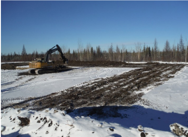
Surface re-contouring of b-008-K/094-I-12 as part of initial reclamation.
