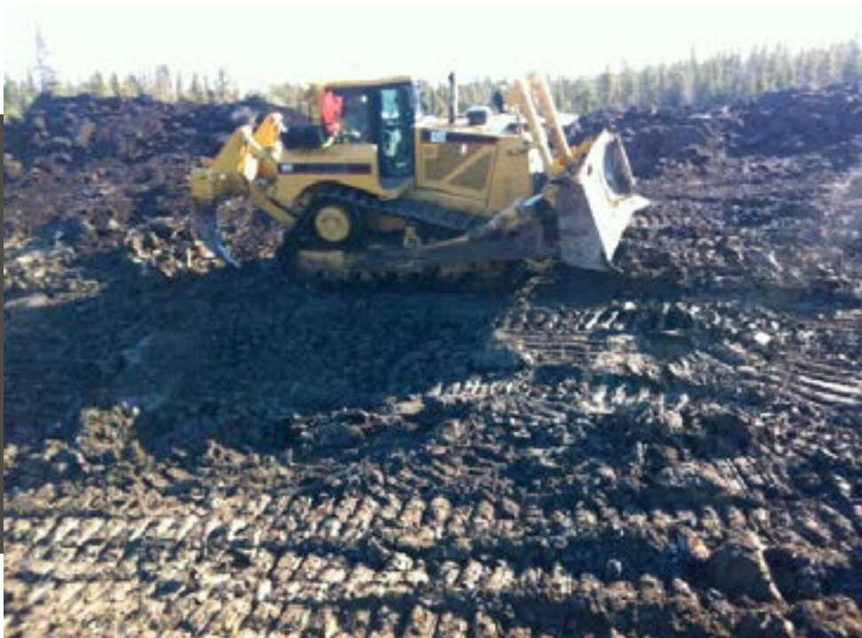
Surface re-contouring of WA# 20634 (c-022-K/094-I-12) as part of initial reclamation.
