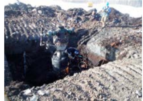
WA# 4343 (b-008-K/094-I-12). Well was plugged in February 2015 and cut and capped (shown above) in March 2015.
