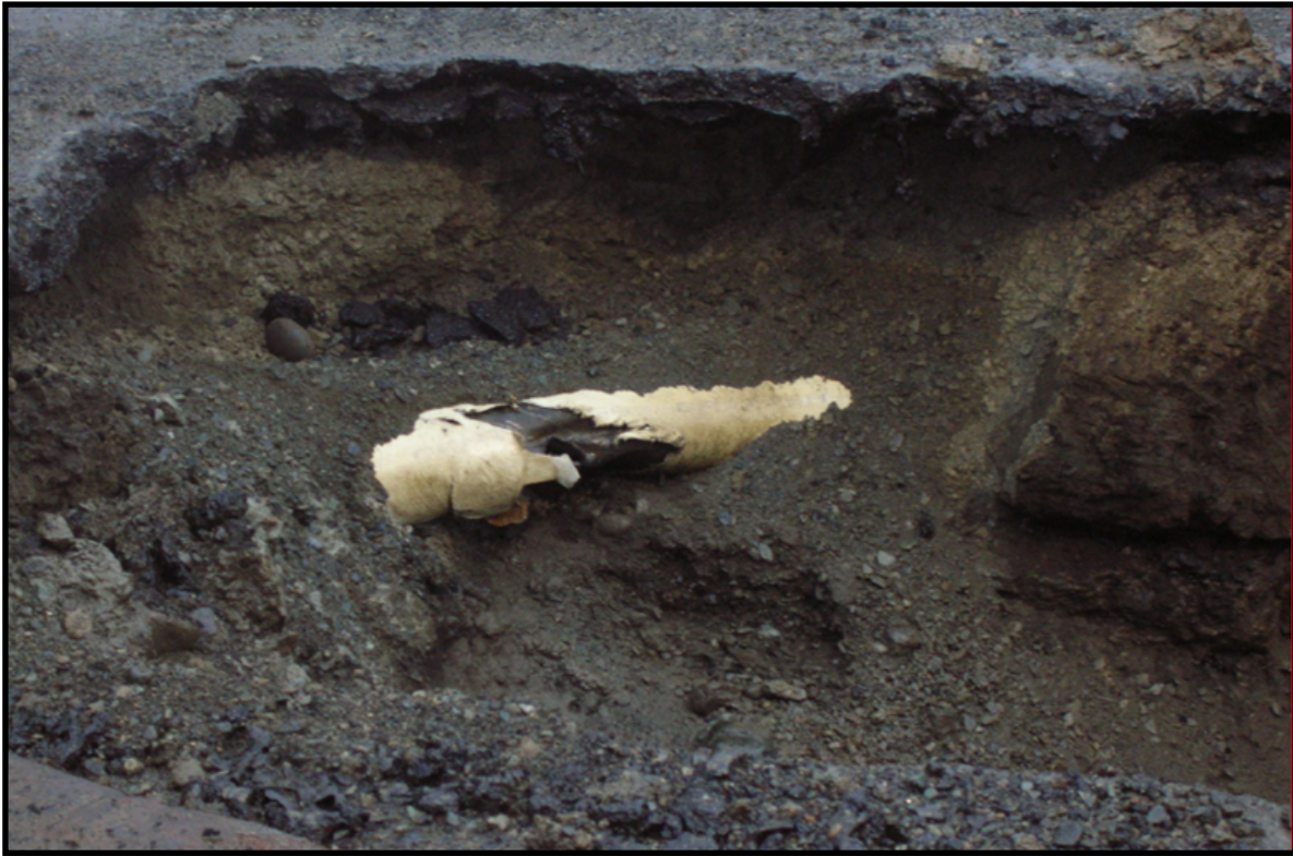
Figure 3 – Damaged Pipe
