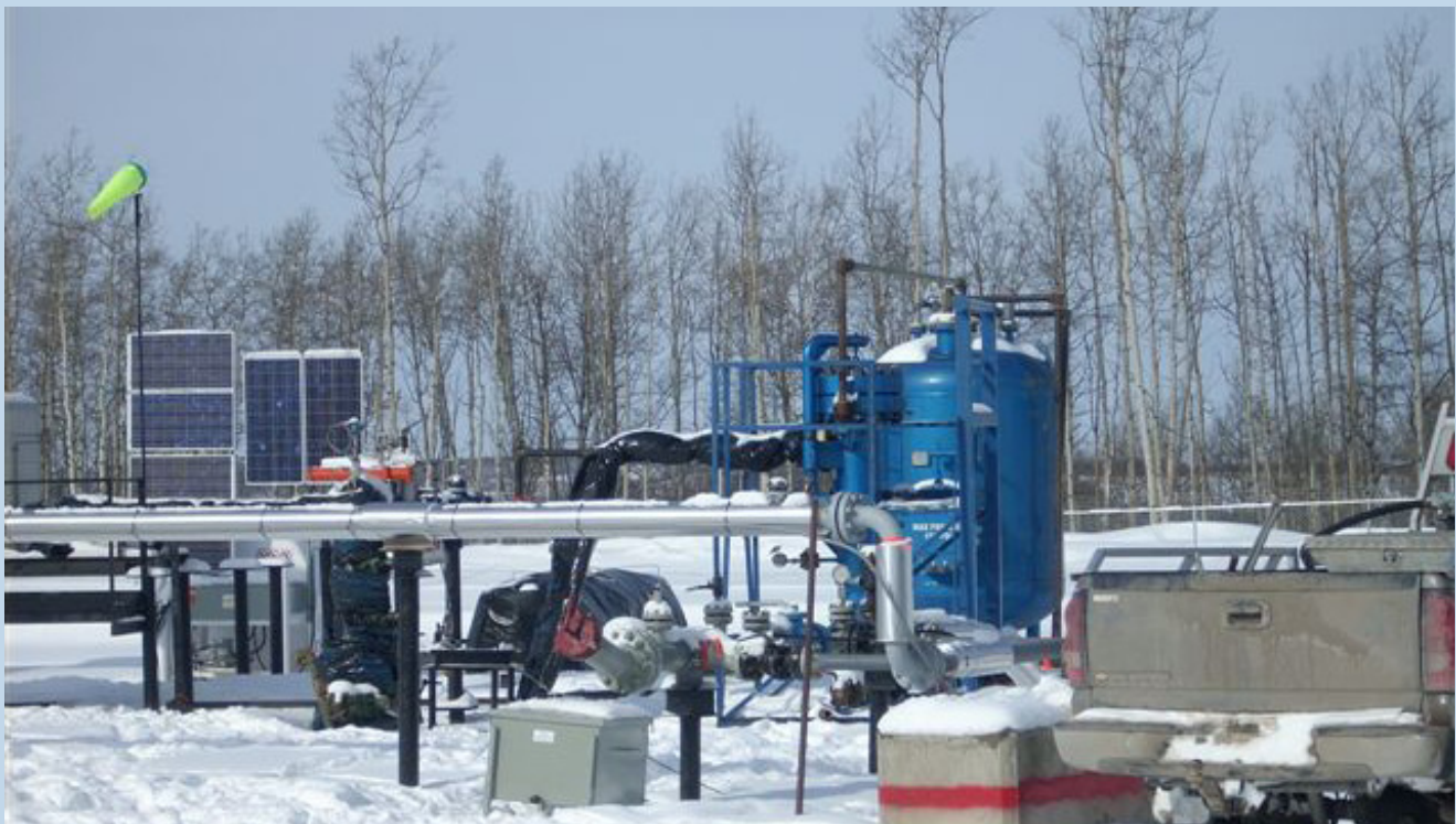
Inline testing at Terra Sunrise utilized for shipping gas through the sales line rather than sending it to flare. A sand filter is used to remove sand from gas. Solar panels harness energy to run both the Scada reporting system and methanol pumps.
