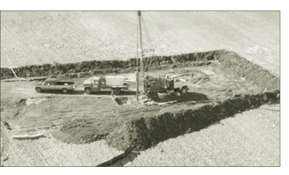
A dirt berm is constructed as a preventive measure in the unlikely event of an uncontrolled release. This is a standard procedure of oil and gas drilling operations throughout the province, and was used as part of CBM exploration. Photo by Boomer Jerritt, courtesy of Priority Ventures Ltd.
