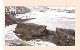
Dam slope failure with no damage to public infrastructure or private property structures, no long- term damage to fish habitat, minimal risk to public safety.
