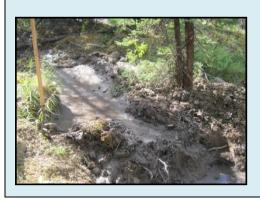
Horizontal boring release of drilling mud to surface, approximately 10M<sup>3</sup>; within ROW
