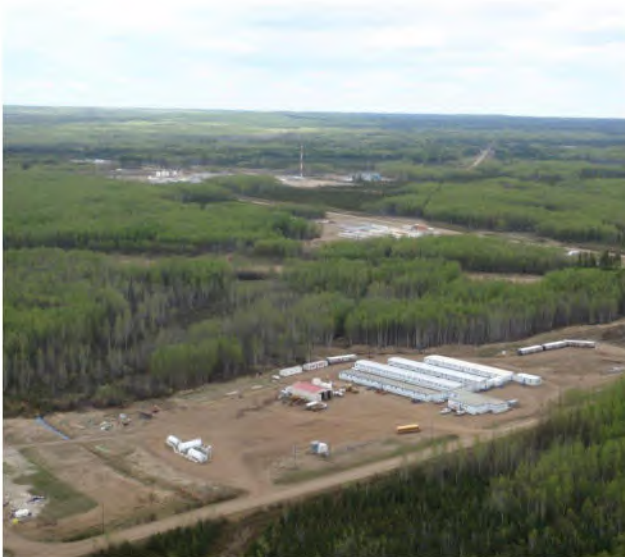
Example of contractor yard and construction camp
