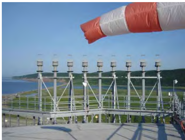
Figure 10 Example of LNG Tank Pressure Relief Valve
