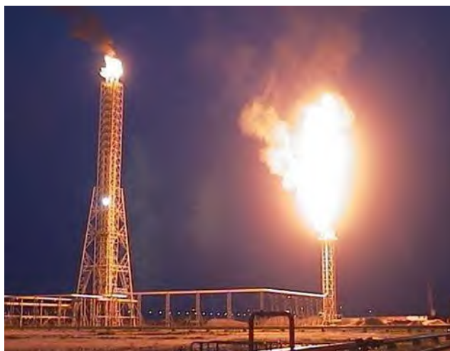
Figure 18 Example of Liquid Burners at night in final cool down
