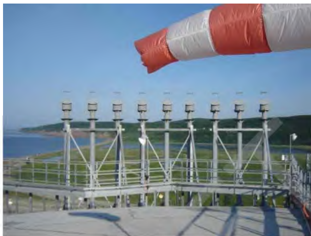
Figure 10 Example of LNG Tank Pressure Relief Valve
