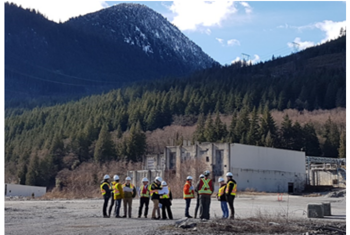
MEMBERS OF THE MAJOR PROJECTS TEAM TOUR THE WOODFIBRE LNG SITE. PHOTO TAKEN PRIOR TO MANDATORY MASK REQUIREMENTS.
