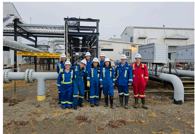
BCER staff at the Aitken Creek Gas Storage Project.
