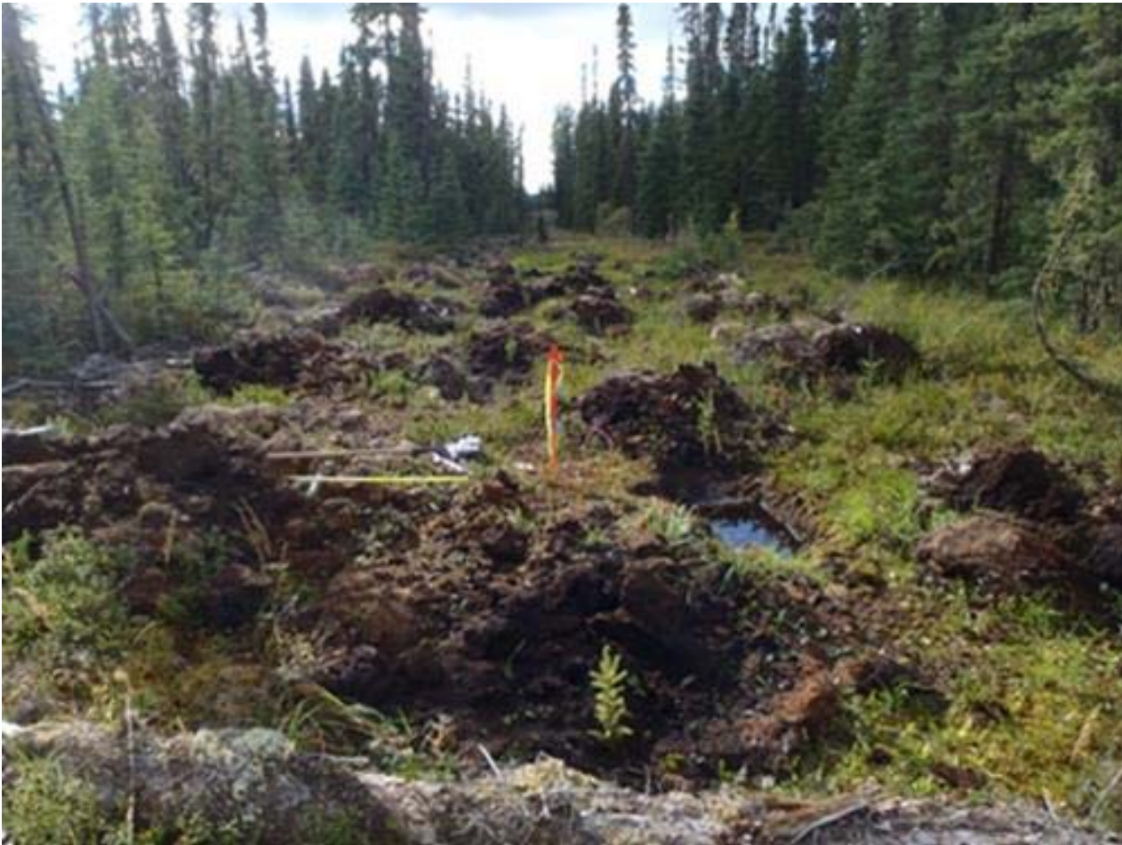
Mounding site preparation is used to recreate hump and hollow terrain features. Benefits are desirable wetland condition and high plant diversity.
