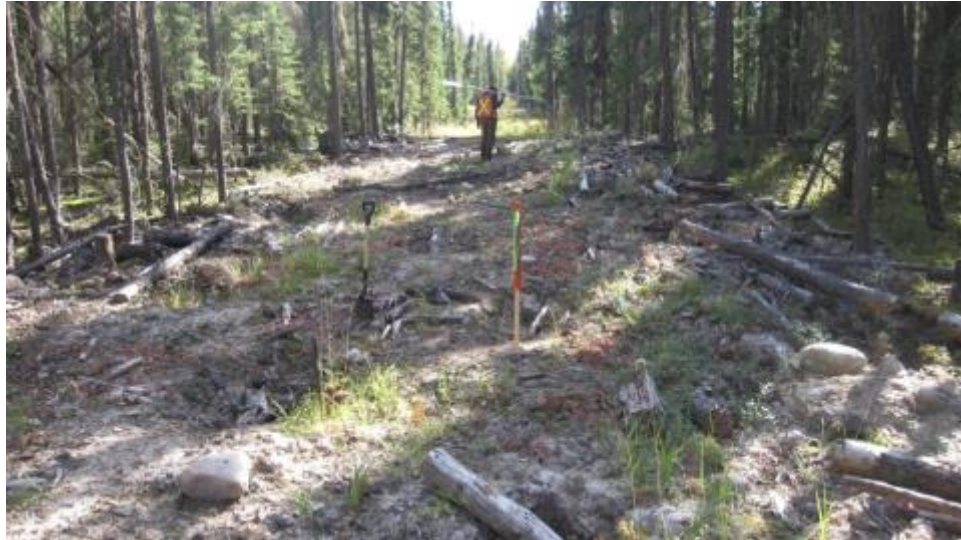
Photo 6: Excavator Ripping in an upland site. (Photo courtesy of Canadian Natural Resources Ltd.)
