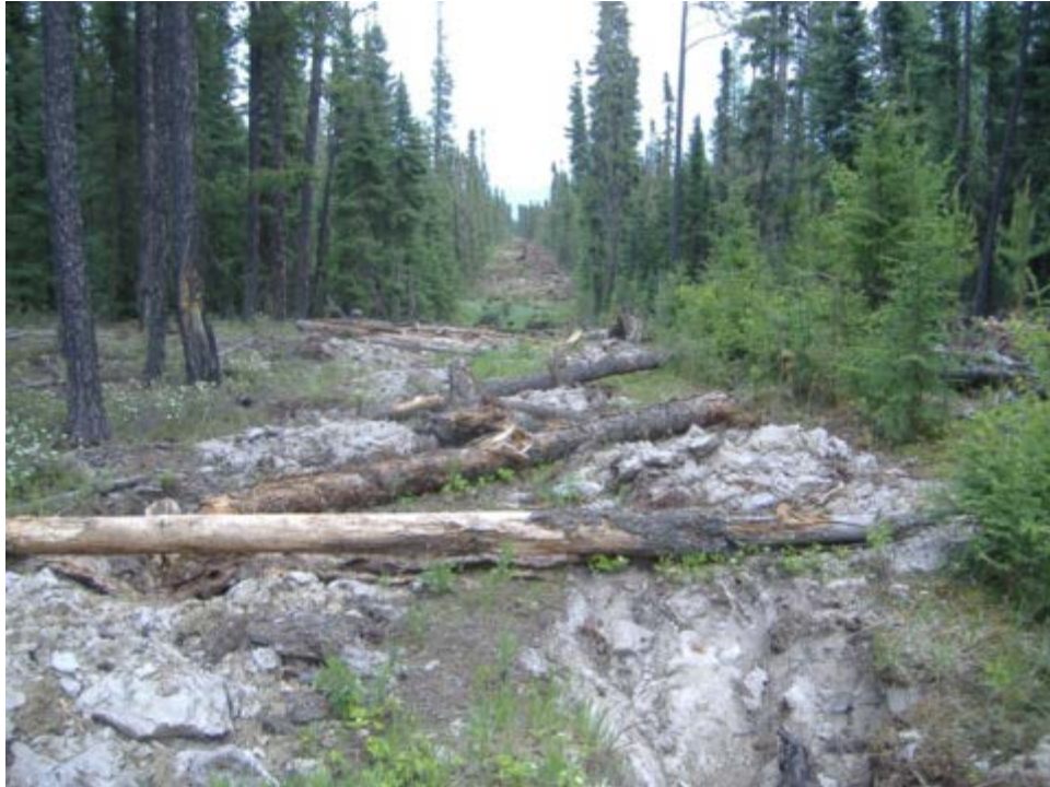
Photo 9: Typical site after undergoing woody material spreading and ripping / mounding treatment. (Photo courtesy of Canadian Natural Resources Ltd.)
