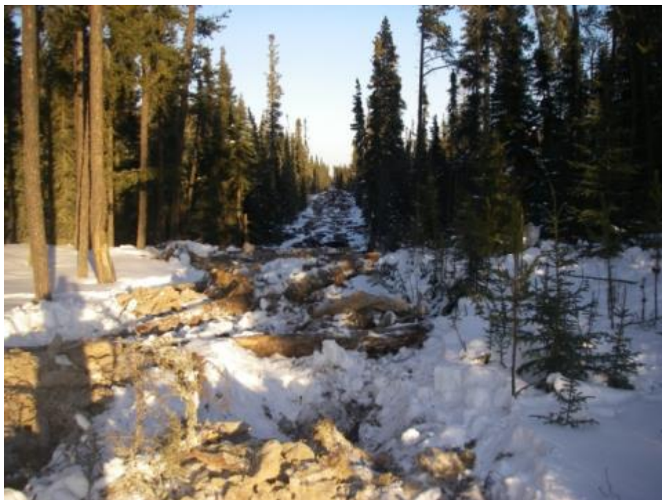
Photo 3: Post treatment in upland site following excavator mounding. (Photo courtesy of Canadian Natural Resources Ltd.)
