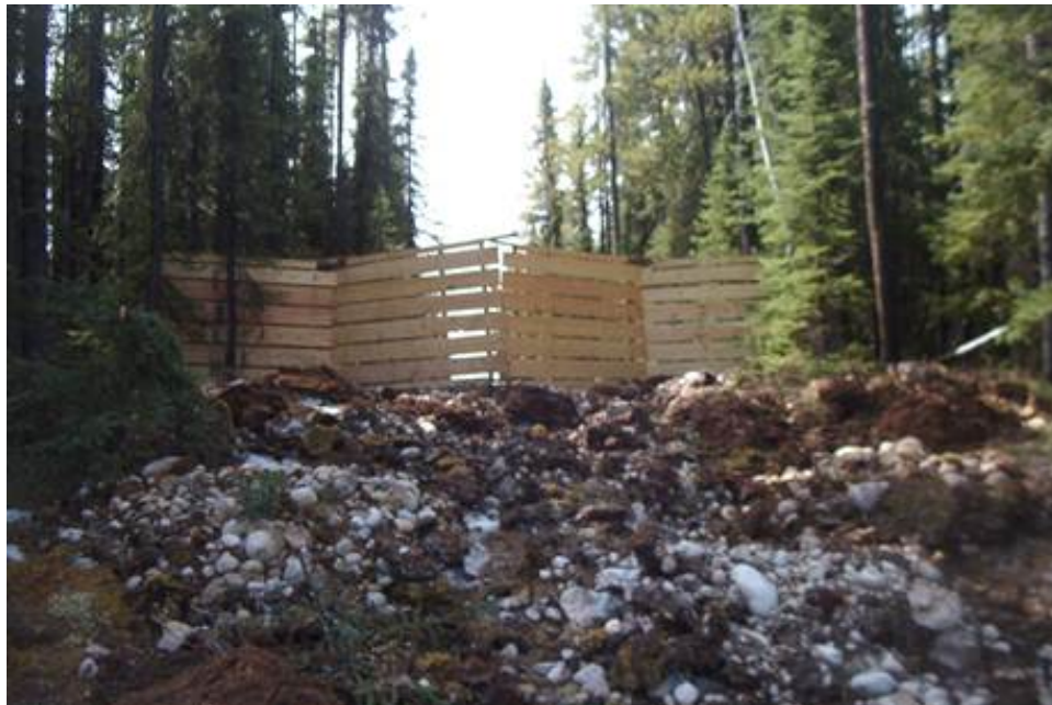
Photo 15: Wooden fence created from panels and installed on a narrow site on the linear feature. (Photo courtesy of Brian Coupal)
